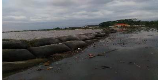
Coastal embankment with sediment/sand trap system
