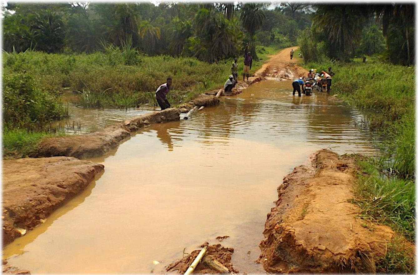
Figure 11: Broken bridge due to flooding
