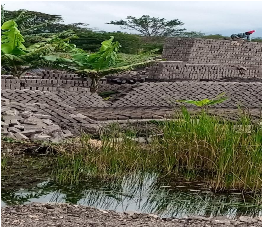
Figure 3: Destructive brick making in the lake buffer zone
