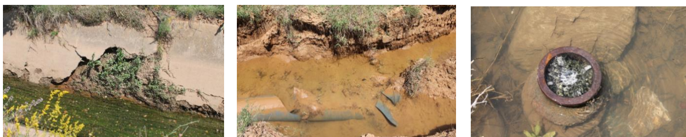
Figure 8: left to right: i) right main channel; ii) burst pipe on the right channel; iii) obsolete flooded hydrant (Source: FAO, 2021)
