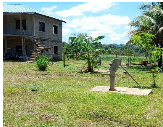
Figure 6: Village Hand Pump for Water (Source: Ministry of Rural Transformation)
