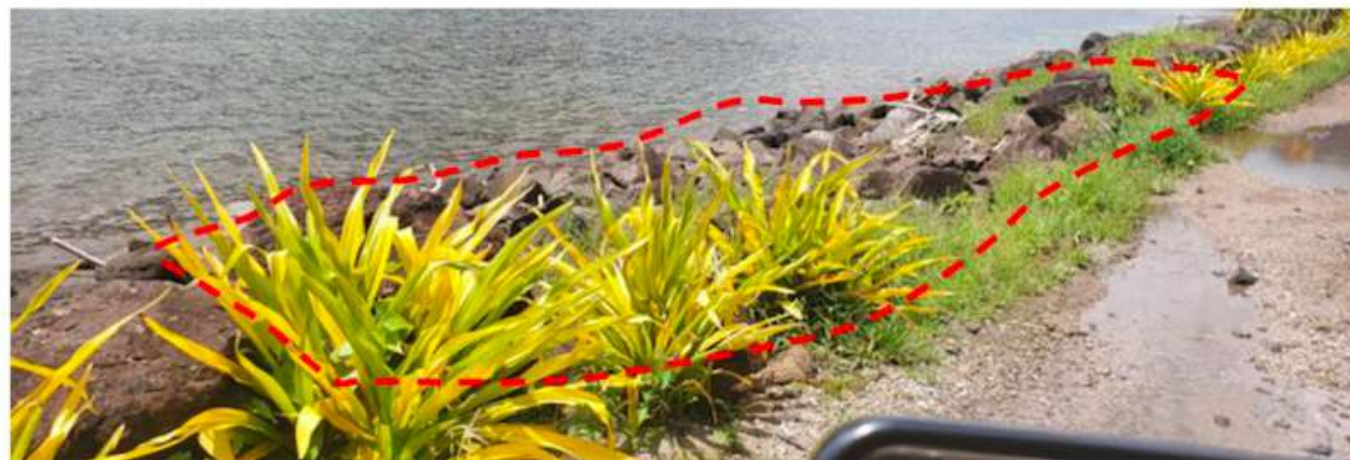
Infrastructure site 4: Salimu/ Musumusu rockwall - Rock undermine from wetland and stream runoff onto the road
