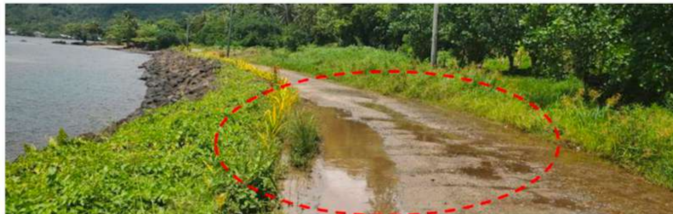
Infrastructure site 4: Salimu/ Musumusu rockwall - Rock undermine from wetland and stream runoff onto the road
