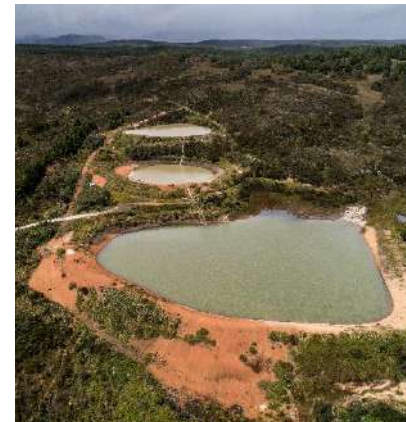
Rehabilitated reservoirs in Cochapata
