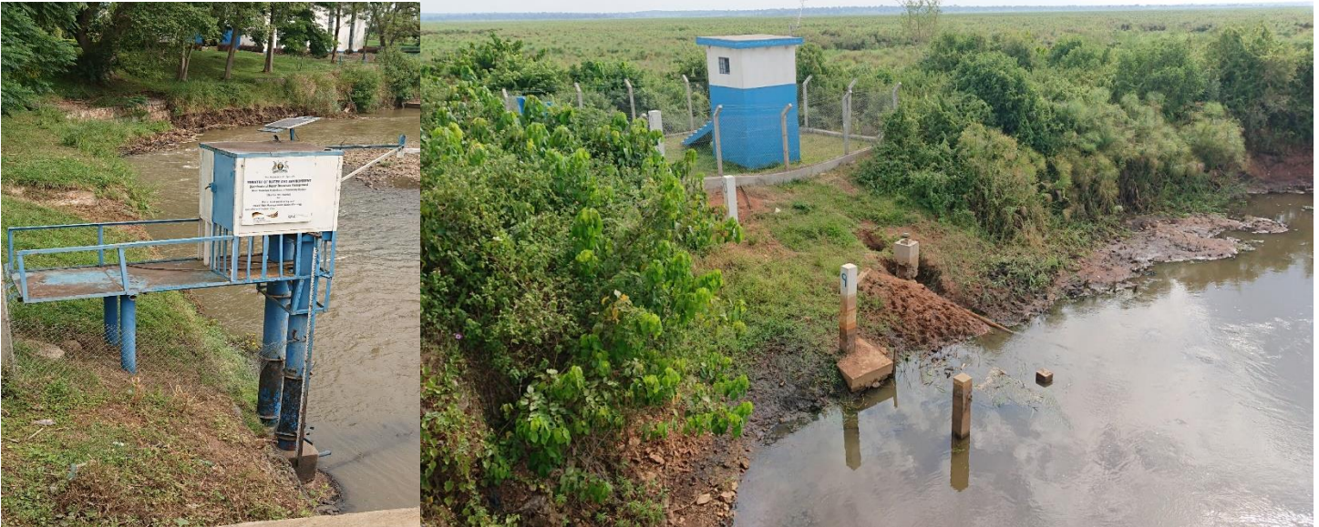
Figure 5: Floods and water level monitoring units at Rivers Manafwa and Mpologoma
