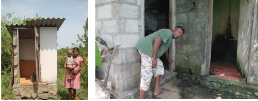
Figure 10: Toilets in flood-prone areas in Welioya DS Division
