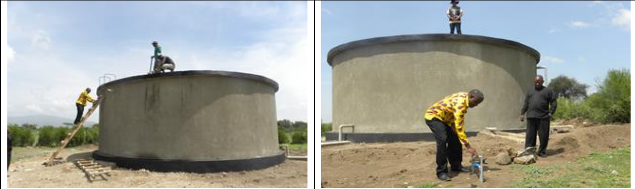
Water storage tank constructed at Meseranijuu Village through a decentralized climate funds.
