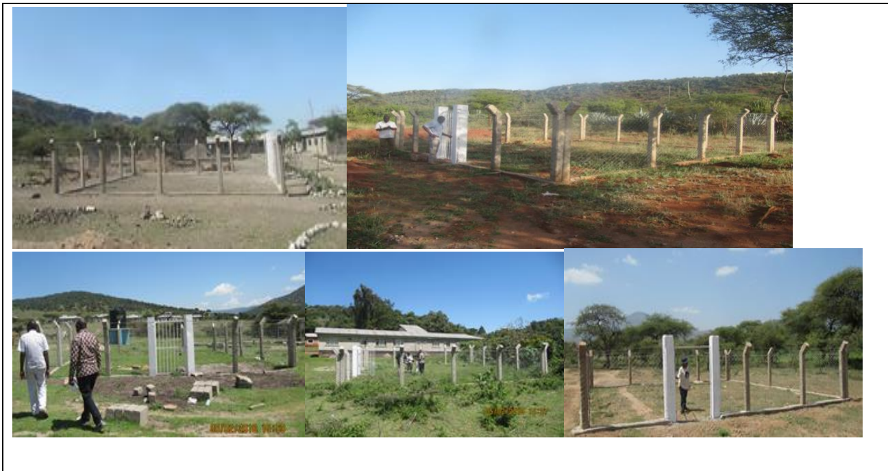
The Installed Meteorological Stations at Ngaresero Primary School, Digodigo Secondary School, district Council Headquarter, Ololosokuan and Malambo.
