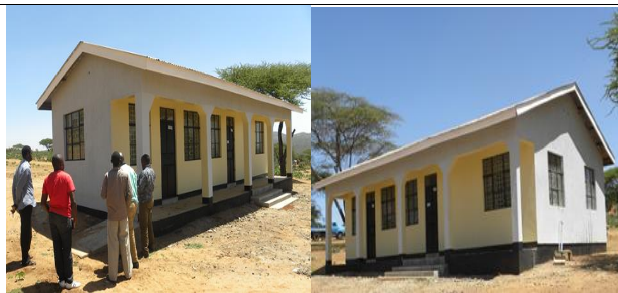
The rehabilitated Mairowa veterinary laboratory.
