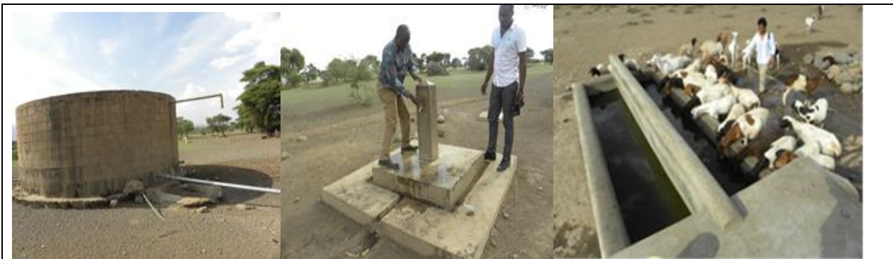
Water storage tank, water delivery points (DPs) and cattle trough in Irerendeni Village, Engaruka
