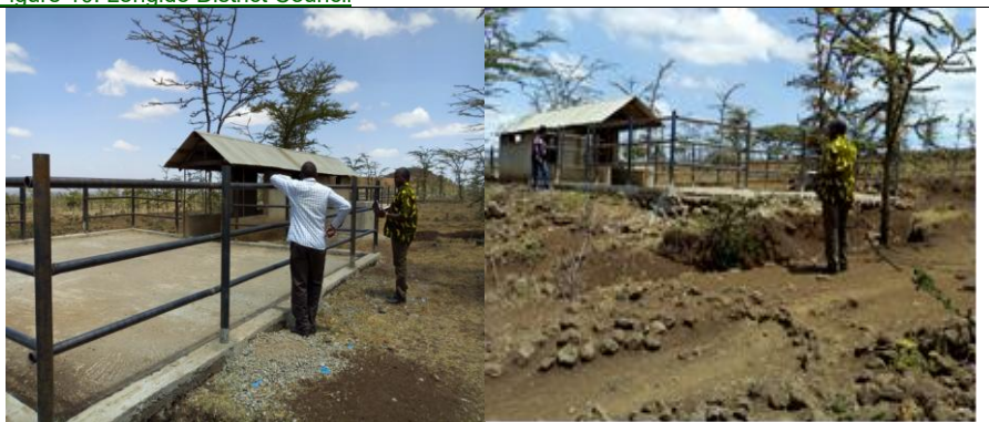
Rehabilitated cattle dip in Lerangwa village.
