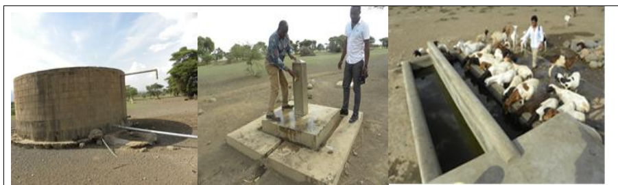
Water storage tank, water delivery points (DPs) and cattle trough in Irerendeni Village, Engaruka
