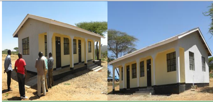
The rehabilitated Mairowa veterinary laboratory.
