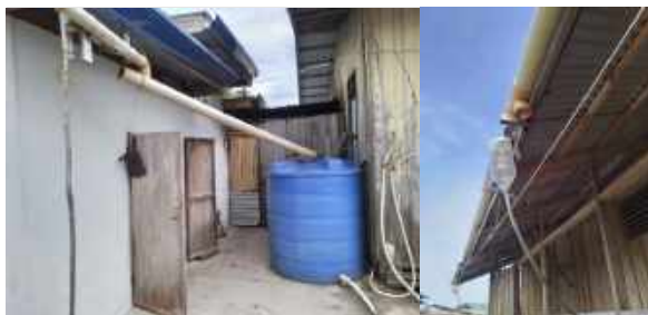
Figure 5. Existing rainwater harvesting systems, Sitangkai
