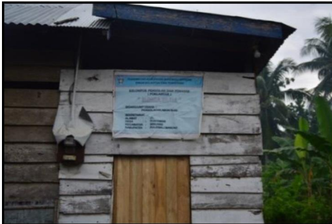
Figure 7 Condition of Silele Flower Group Production House 8
