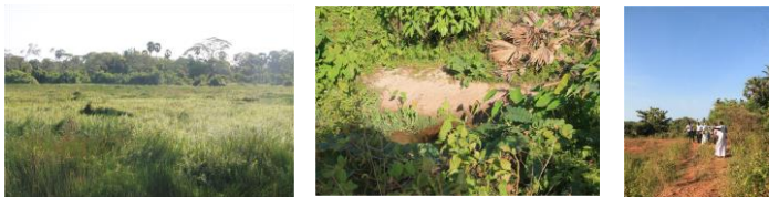
Figure 7: Irrigation tanks and channels (to be renovated) with overgrown grasses and bushes in Mulliyawalai GN Division in Maritimpeattu DS Division
