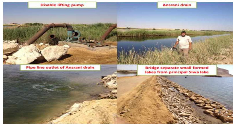
Figure 6: Water Drainage and stagnation issues
