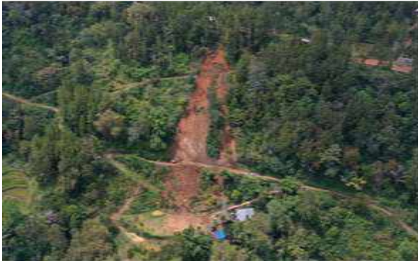
Figure 2. Landslide in the upstream Saddang watershed, 2021 (Doc: Kemitraan-TLKM)
