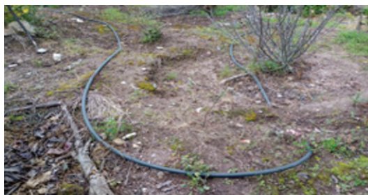
FIGURE 2: Abandoned garden with piping, Nabón
