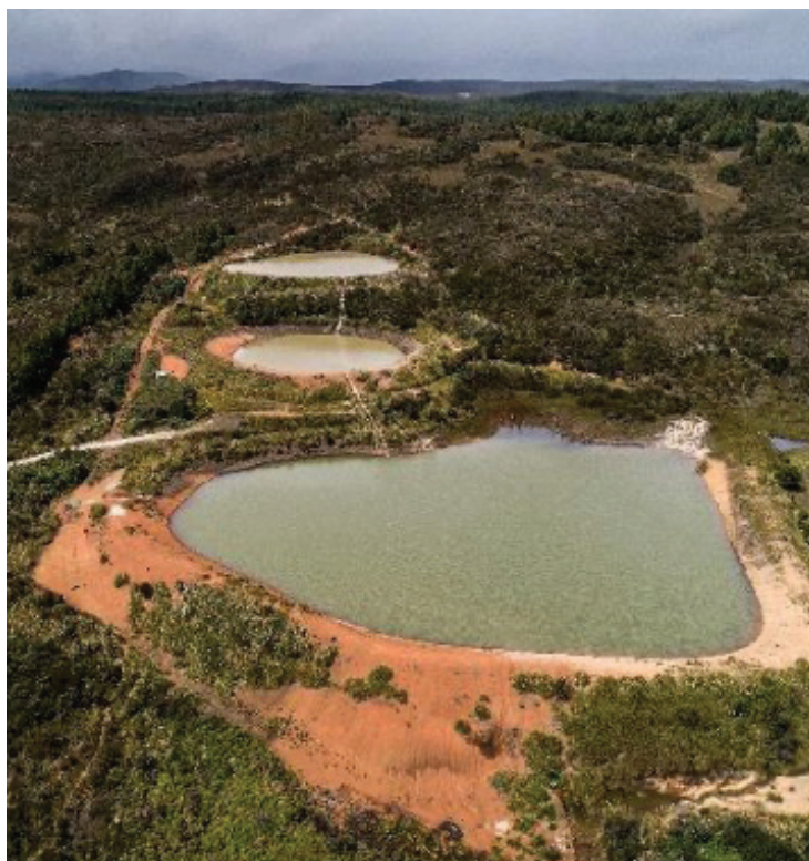
FIGURE 3: Rehabilitated reservoirs in Cochapata
