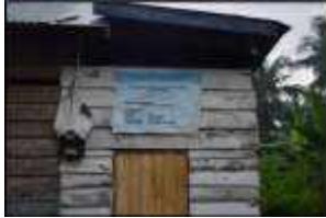
Figure 7 Condition of Silele Flower Group Production House 6
