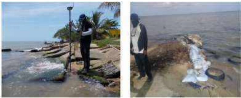
Figure x. (left) Destruction of the facility by erosion in Dangriga. (right) Type of ineffective defense structure Figure 16: (left) Destruction of the facility by erosion in Dangriga. (right) Type of ineffective defense structure.
