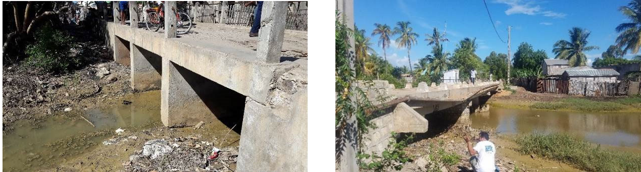
Figure 8: Bridges crossing the Hellot Channel
