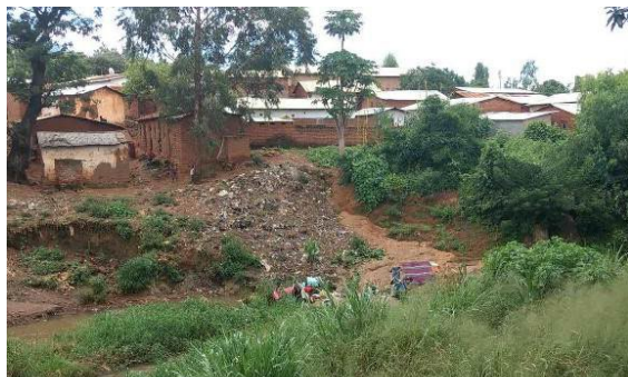
Figure 14: Encroachment of settlements near the Likangala River
