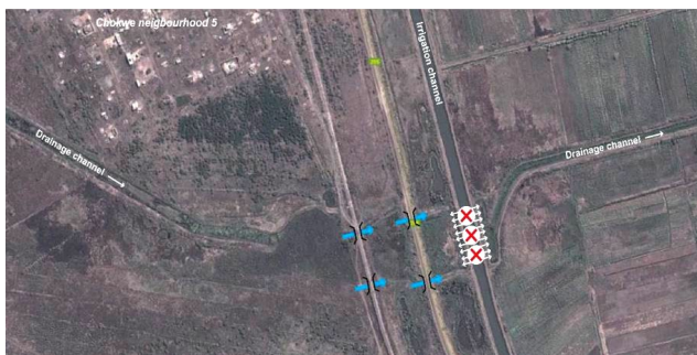
Figure 20: Detail of crossing "2" where the pipes under the irrigation channel are collapsed
