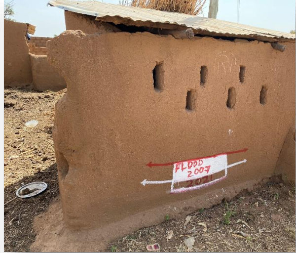
Flood water level markings are an important element of warning residents when they must evacuate their homes.
