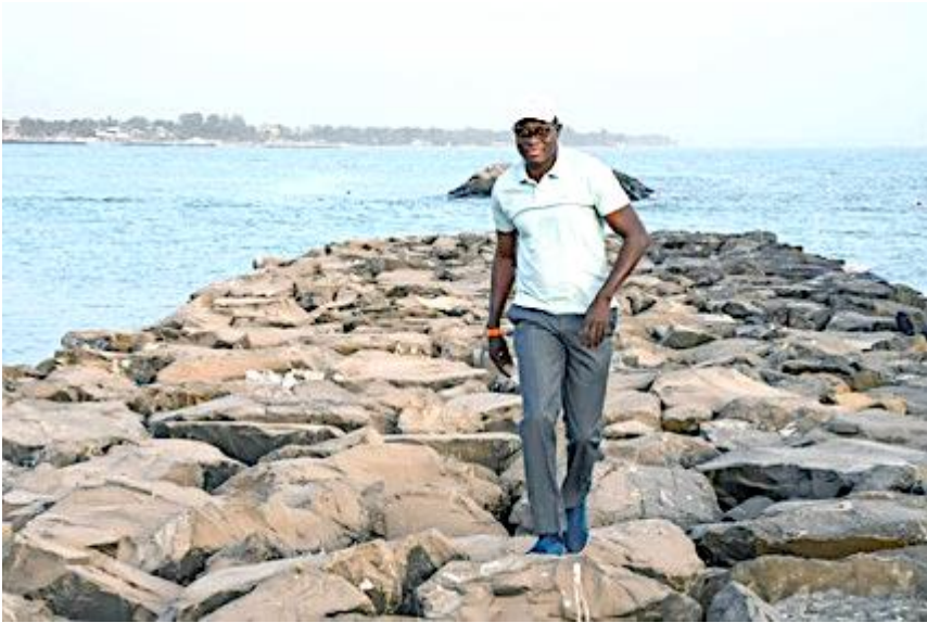
Breakwater of Saly Portudal (Senegal))
