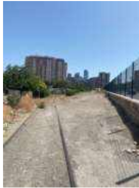
Image A.1-4: Cement coverage along the former railway line
