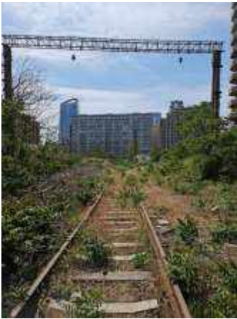
Figure 27: In the background, an older and rundown residential block, visible also in the bird's eye view below (*).
