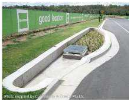
Figure 54: Component of a drainage system
