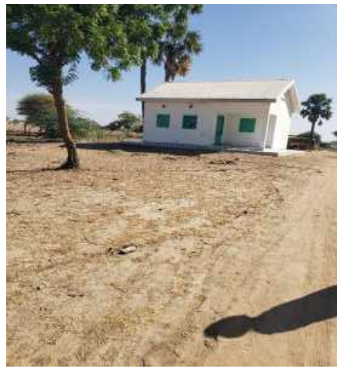
Hydromet station housing Kousseri
