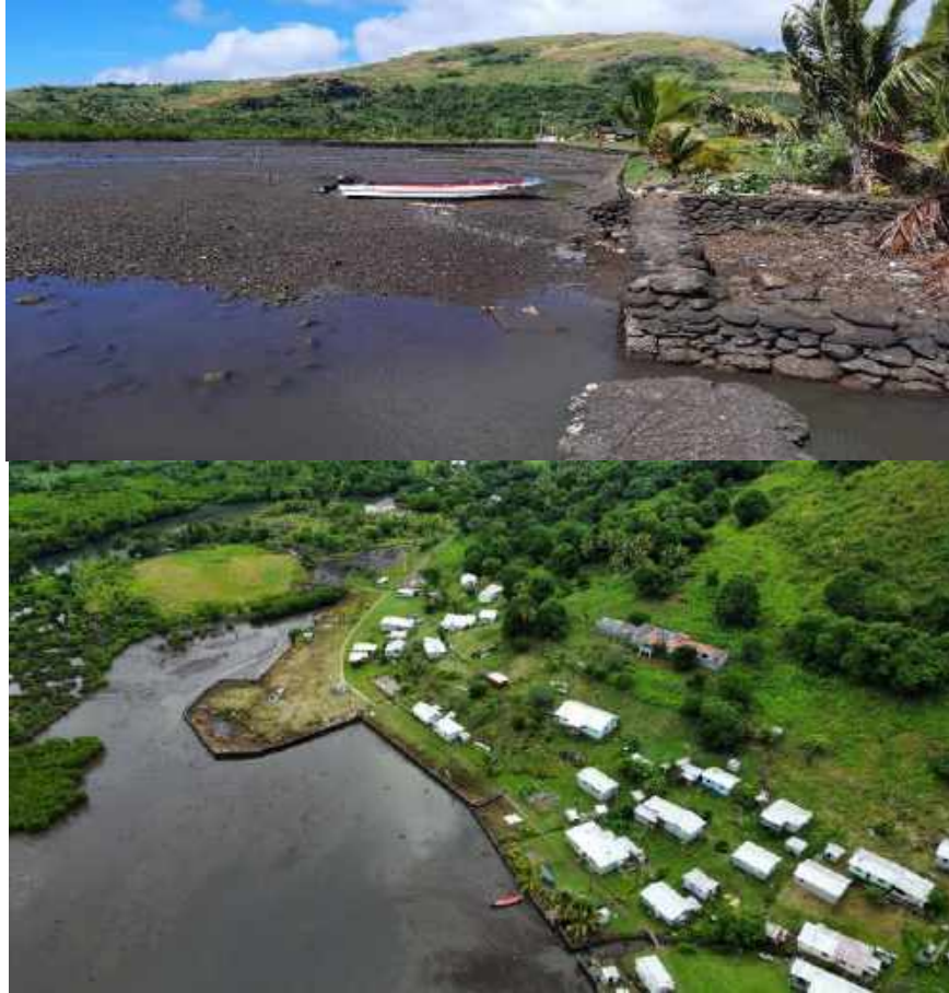
Figure 402: Project site at Nayavutoka Village
