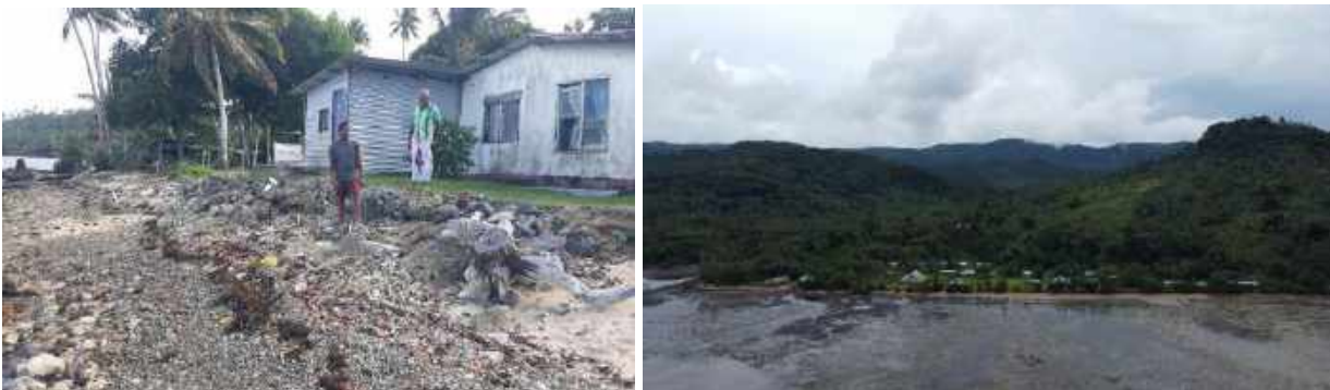
Figure 30: Project site at Sese Village
