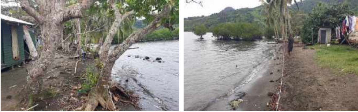
Figure 34: Project site at Loa Village
