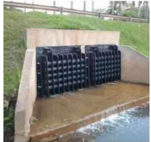
Figure 2 – Example of Flap Gate - FLOGATE HDPE, link
