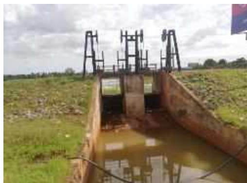
Figure 5 Outlet structure
