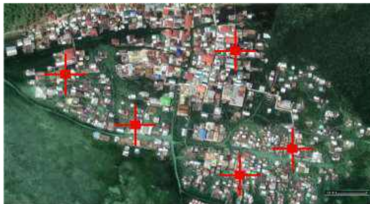
Figure 4.12. Illustrative example of a web-like network of shared communal sanitation system with a cluster of households along canals or foot bridges.
