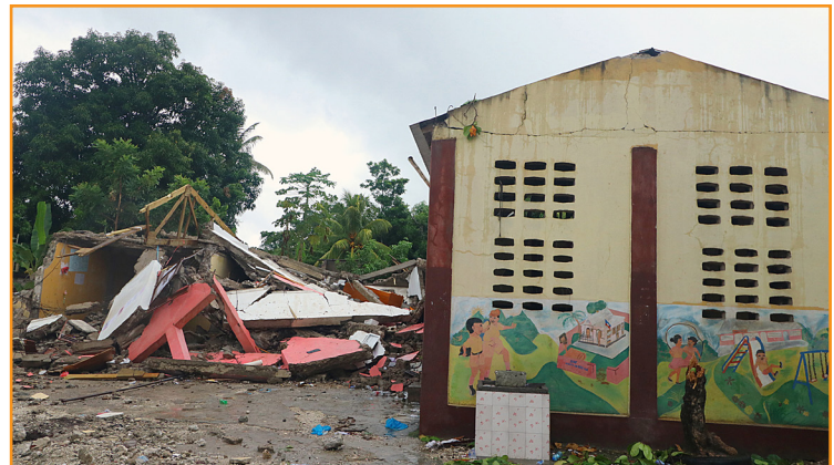
Schools damaged in L'Azile, borough of Miragoâne, geographic department of Nippes during the earthquake of August 14, 2021 in Haiti. (Photo: UNESCO)
