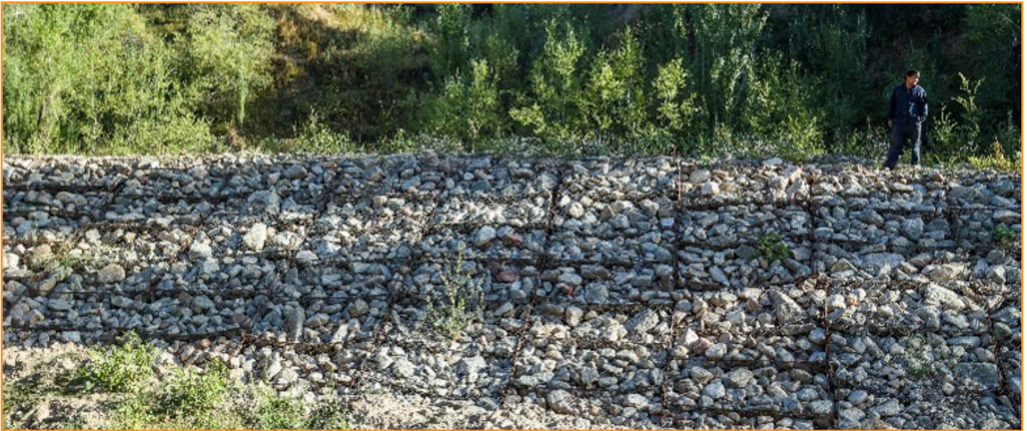
Manuchehr Makhmudov, a 34-year-old resident of Boboi Vali village of Fayzobod district, is standing on a stone fence to prevent erosion, as part of the project. (Photo: UN Development Programme)
