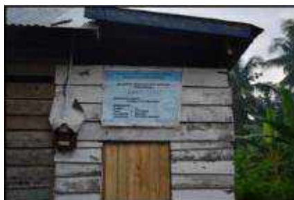
Figure 7 Condition of Silele Flower Group Production House 6
