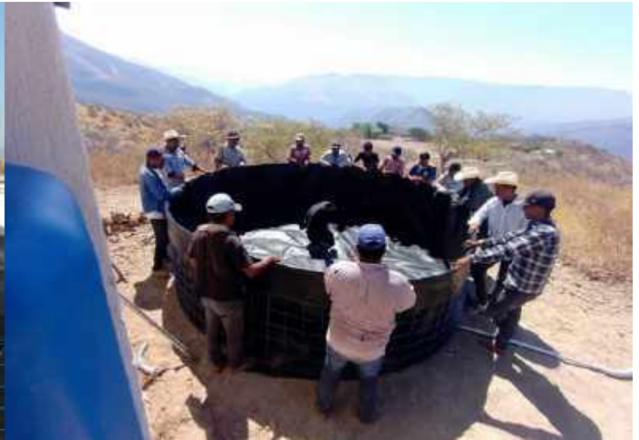
Participative cistern installation
