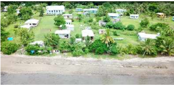
Figure 46 Site for NbS seawall installation in Nabuna Village
