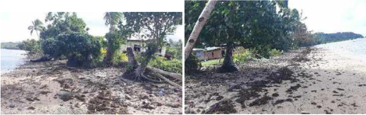
Figure 30: Project site at Saqani Village
