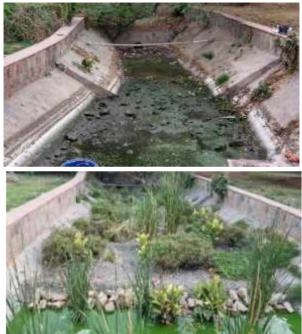
Figure 10 – Outfalls Conversion of a drainage canal into a subsurface flow constructed wetland
