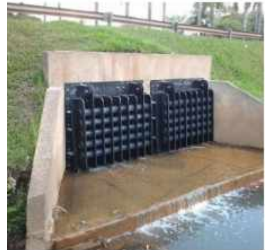
Figure 2 – Example of Flap Gate - FLOGATE HDPE, link
