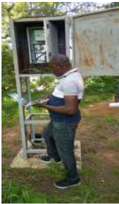
Hydromet Station (CHAD)
