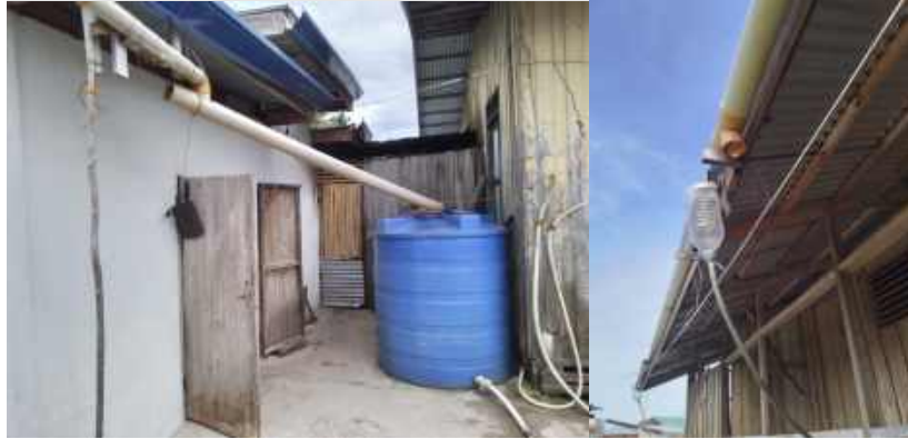
Figure 5. Existing rainwater harvesting systems, Sitangkai
