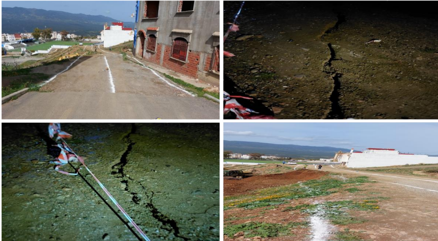
Fig 5. Example of areas at risk of landslides in the Municipality of Chefchaouen (Ain Haouzi neighborhood)
