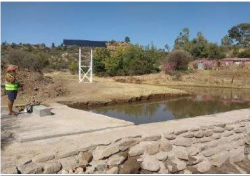
Figure. A7.1: Sand dam built in 2024 at Waterfall in Lesotho, with solar pump
