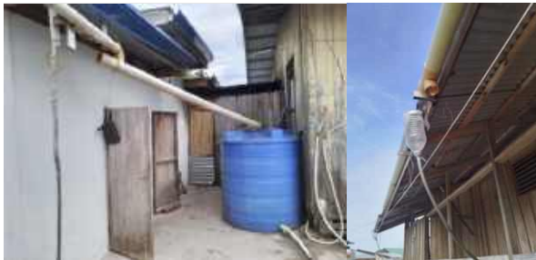
Figure 5. Existing rainwater harvesting systems, Sitangkai
