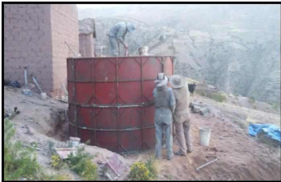
Photo 7. Concrete storage tank require a special mold with a tailored design to this technology, the program proposes creating its own molds for the sustainability of the project
