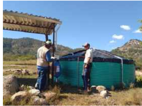
Photo 5. RWH system with metal sheet protection
