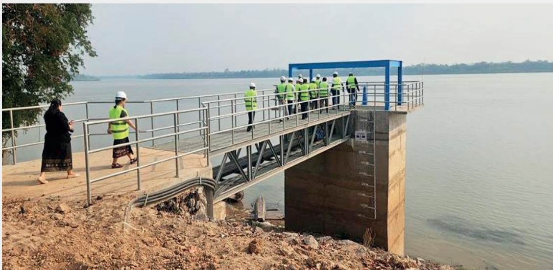
Figure 3 – Intake structure for water treatment plant (WTP) in Sayphouthong
