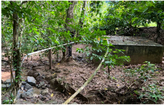
Figure 35: Spring Water Reservoirs with PVC Pipes to the Village (Source: Site visit 2023).
