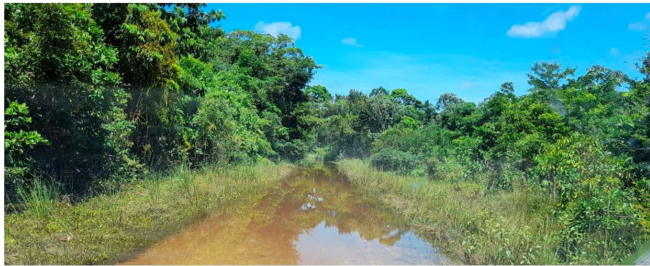
Figure 28: Boom Creek Road during flooding (Source: Boom Creek Village Needs and Assets Assessment, 2021).
