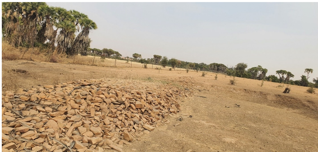
Figure 10. Water retention stone cordon in Leweinatt with protected grazing area in the background
