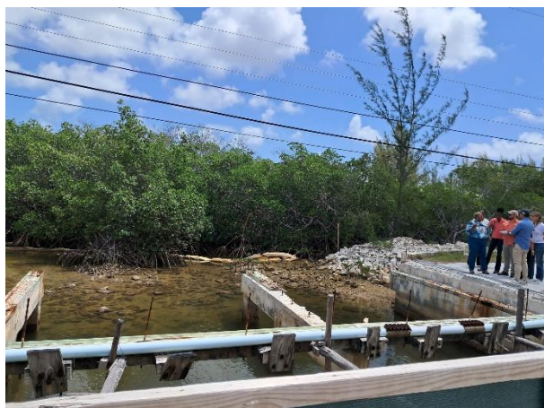
FIGURE 6. DAVEY CREEK BRIDGE
