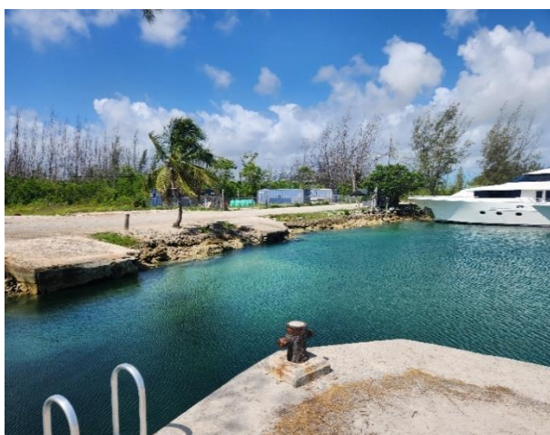
FIGURE 4. THE BOAT RAMPS AT MORGAN'S BLUFF
