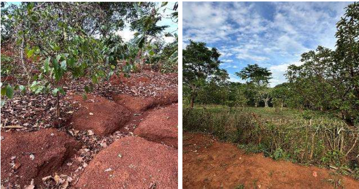
Figure 19: Drainage channels in coffee garden and agroforestry in Kaliro district
