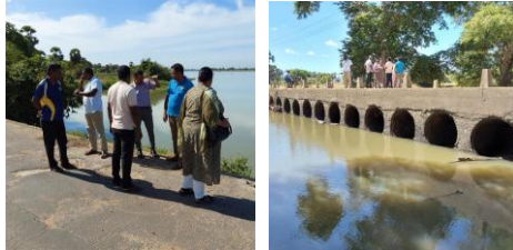
Figure 8- Site inspection to a local culvert. Source: UN-Habitat field visits
