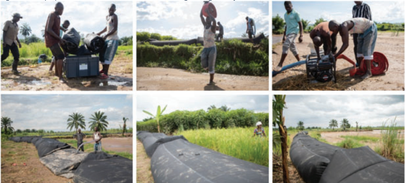
Figure 1 Dual-purpose mobile flood barrier and water storage & irrigation system
