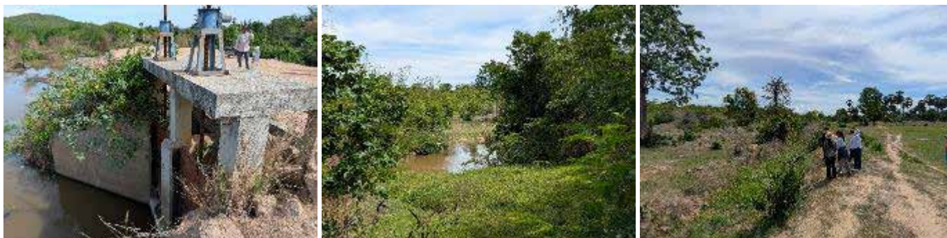
Figure 2. Existing water gate/sluice (left), canal with vegetations (middle), and small field channels with sediments and vegetation (right)
