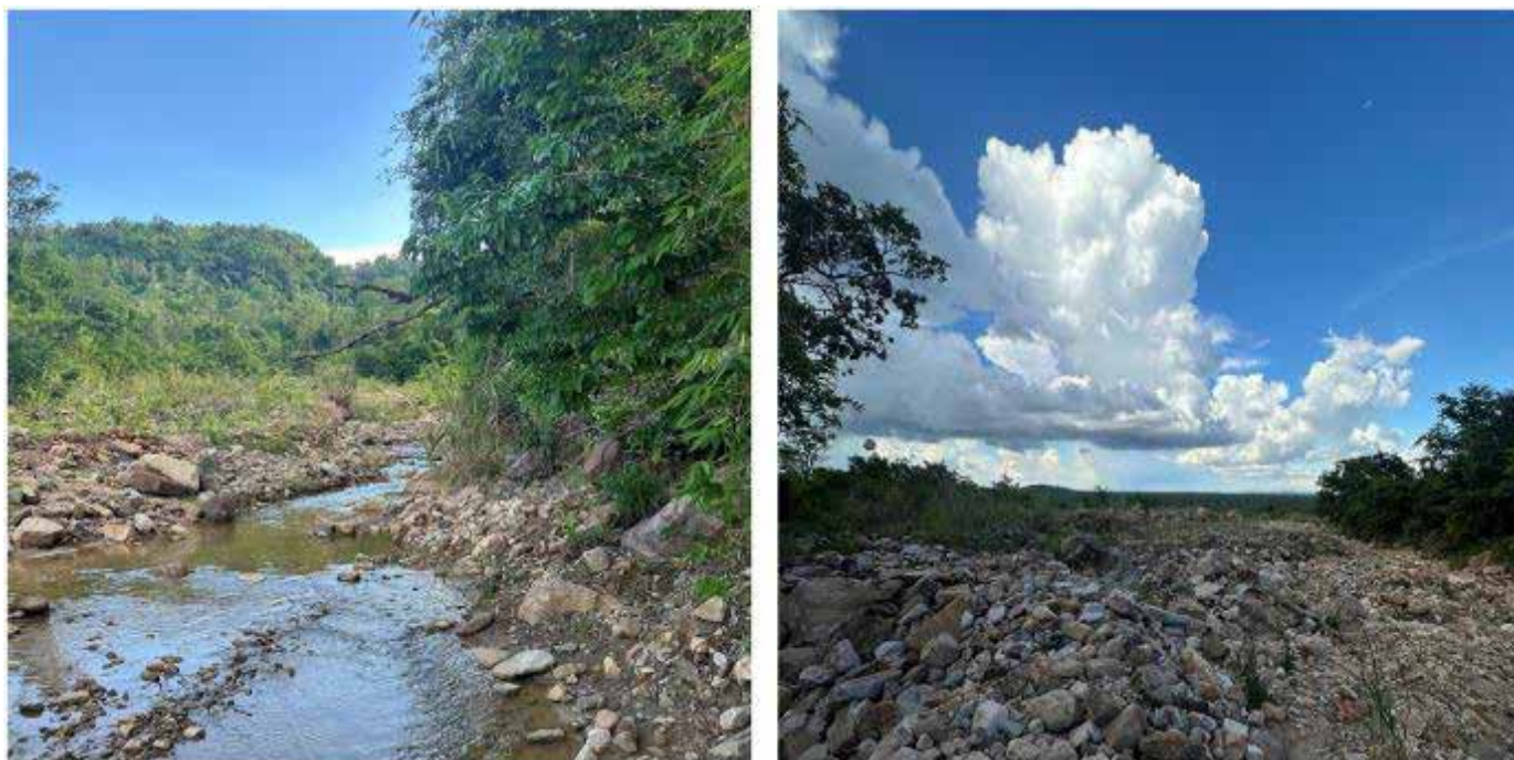
Figure 2. Existing situation of the site for a new rock dam (left) and irrigation canal rehabilitation (right)
