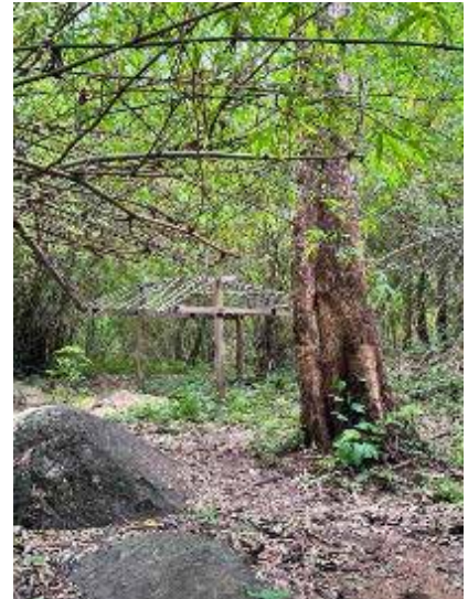
Figure 9. Example of a simple existing structure beside the trail that could be adapted and used as a rest area.
