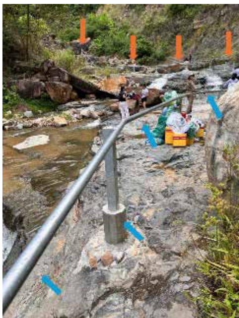
Figure 2. Existing handrail configuration and proposed realignment, relocating the crossing from the riverbed to the left bank to improve safety, flow continuity, and landscape integration. Orange arrows indicate the proposed alignment, while blue arrows highlight sections to be retained, upgraded, or removed.
