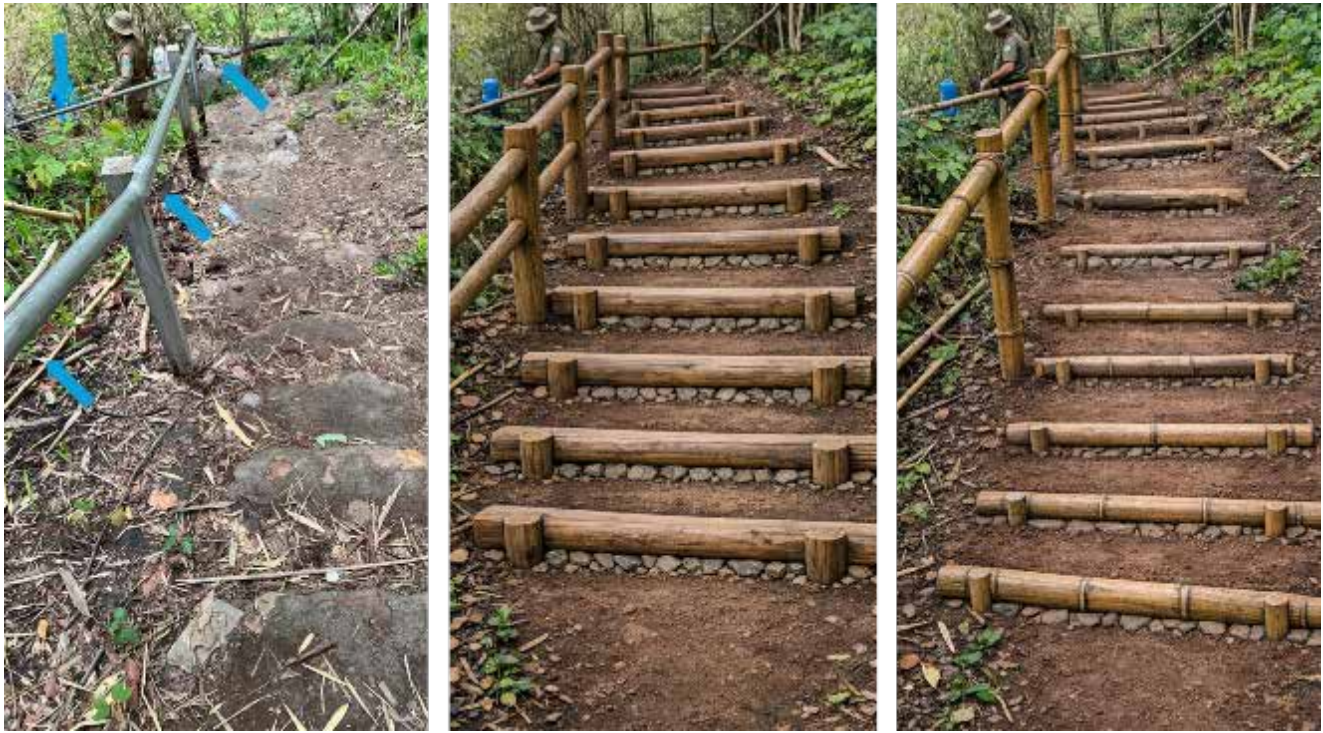
Figure 3. Proposed Nature-based Solutions (NbS) interventions for trail stabilisation, drainage improvement, and safety enhancement in a steep section.
