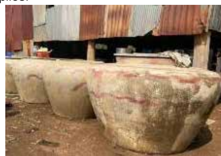
Photo 1 Example of rainwater collection and storage at a household
