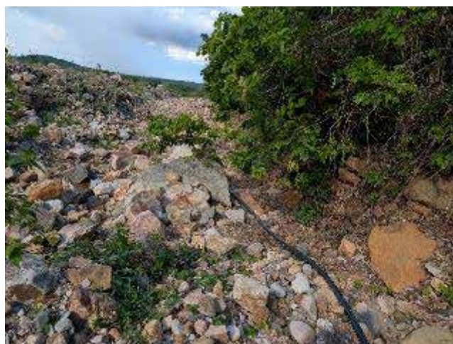
Figure 5. Existing irrigation canal filled with rocks from the previous upstream dam.
