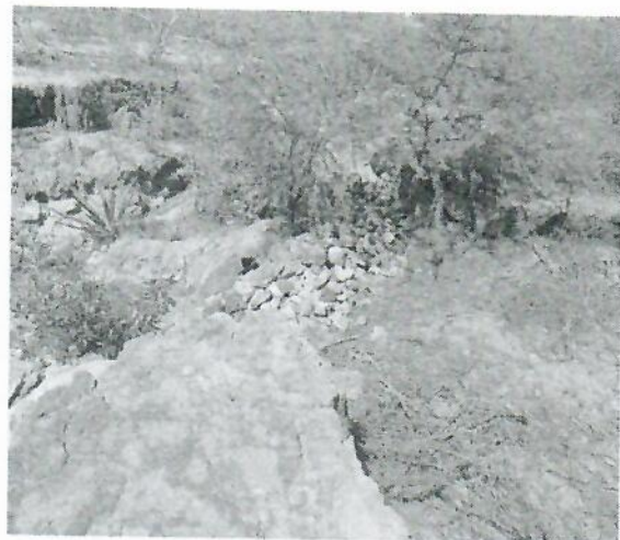
Planting of vegetation and inserting rocks as measures to counter the expanding gully
